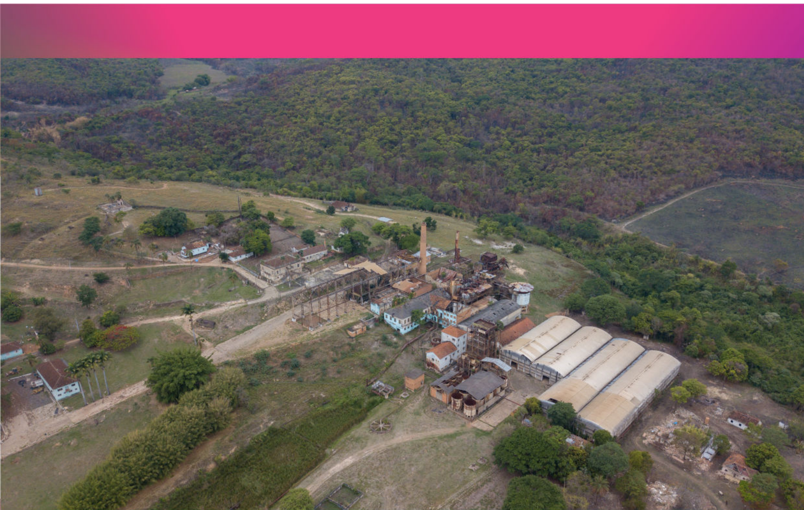
Aerial photo of ruins of the plant that originated the MST occupation in Campo do Meio (MG)
